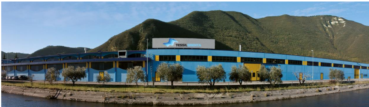
Tessilbrenta S.p.A production plant – Pove del Grappa (VI)
