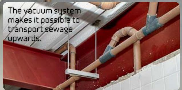
The vacuum system makes it possible to transport sewage upwards.
