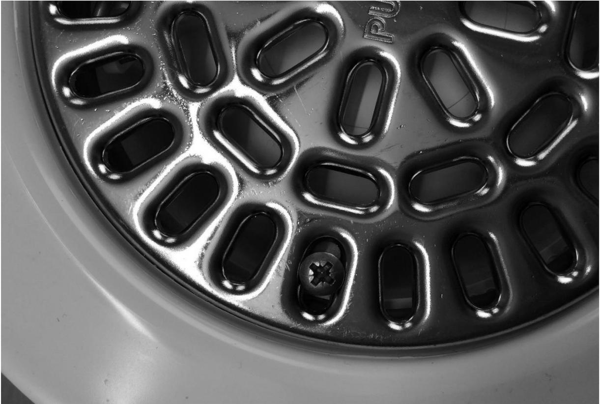
Look thru the grating, there you can see and make sure that the locking clips are fastened under the clamping ring. Take the screwdriver and turn until the grating is in place. A good tip is to screw gently first on one side then the other side, then the first side again. Then you are ready!
