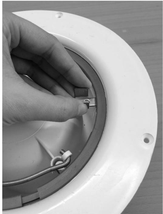
On the locking clip you can see a small flange, this is locking the grating so make sure to get it secured under the clamping ring. Pictures are just to illustrate how they are secured later in the process.
