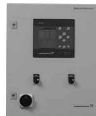
Fig. 4 Grundfos Dedicated Controls
