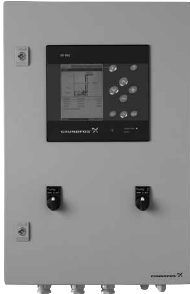
Fig. 38 Dedicated Controls control cabinet
