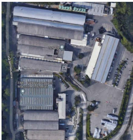
Figure 1: Tenax S.p.A production plant – Viganò (LC)
