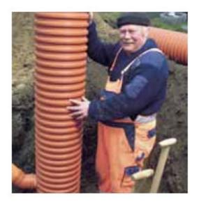
2. Add sand layer to correct chamber invert level. Compact the sand.
