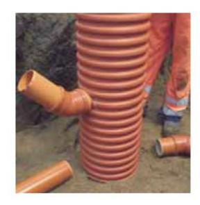
4. Install pipe connections.
