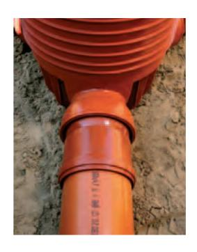
5. Fill the chamber pit with gravel. Compact in layers up to the top according to local regulations.
