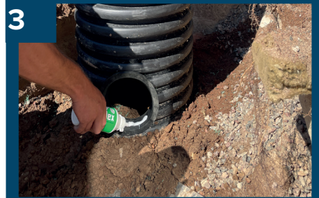
3 Montera packning.
