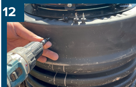
12 Skruva fast locket.
