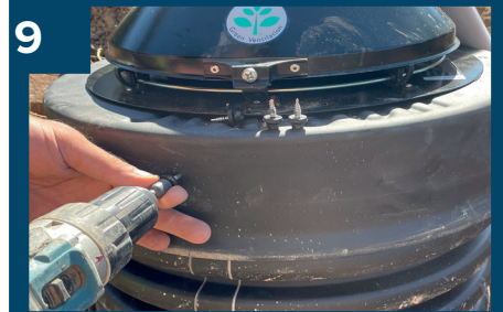
9 Skruva fast locket.
