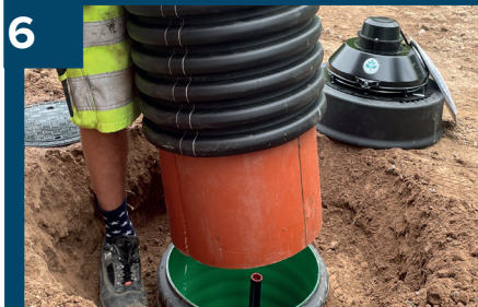
6 Montera teleskop i pumpbrunn.
