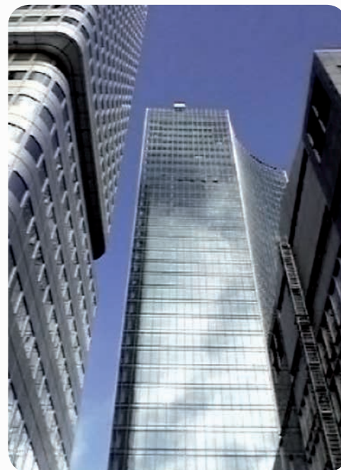
Reference property item – Skyper high-rise offices, Frankfurt a.M.
