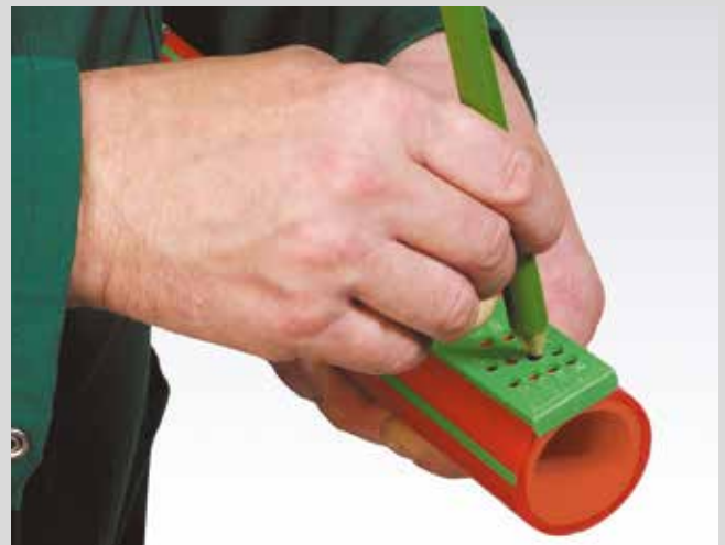
Marking of the welding depth
