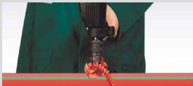
Drilling through the pipe wall
