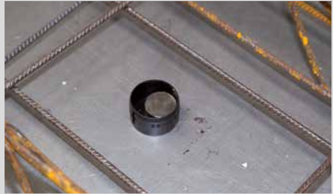
Base part of sprinkler outlet Art. no. 4114180 for visible sprinklers. Attachment by magnet.
