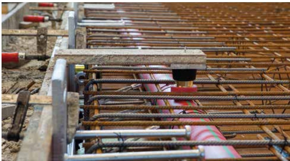
Prefabrication concrete wall
