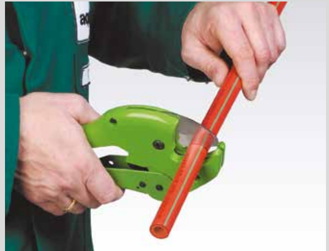
Cutting of the pipe
