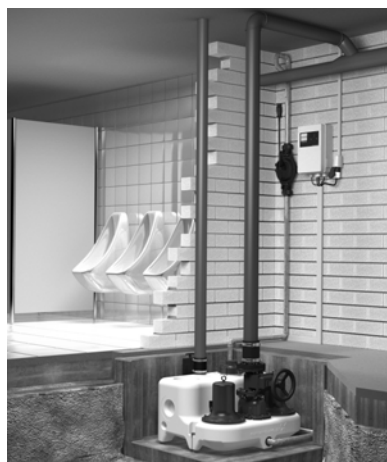
Fig. 27 Example of installation of Multilift MDG in a pit in the building's basement
