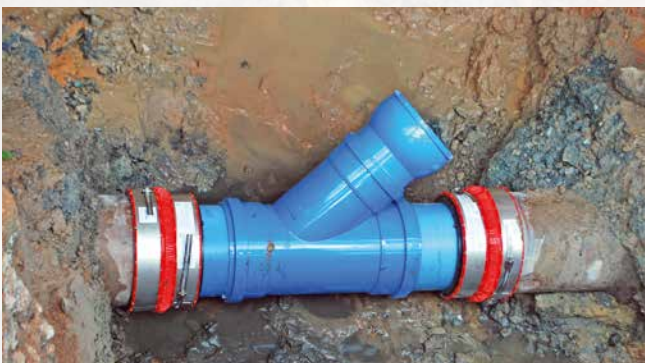
Retrofitting a branch element into an existing vitrified clay pipe
